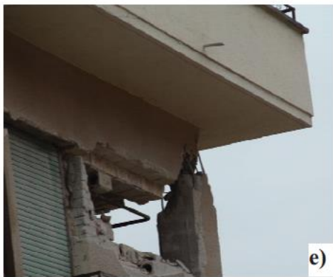
Figure 1. Masonry infill-related damage in recent earthquakes.
